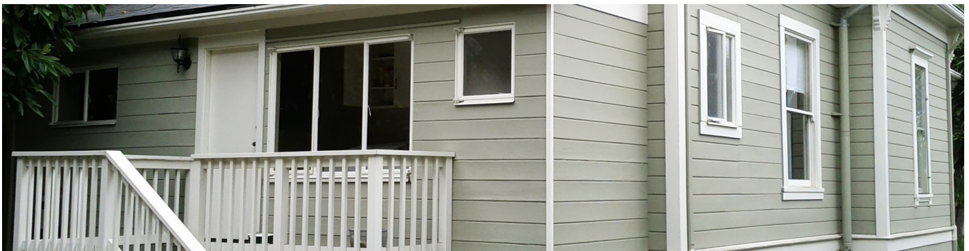
This photo shows three of the steel frame casement windows on the rear addition, as well as one more on the side of the house (nearest the back), in contrast to the original wooden window shown at the far right
