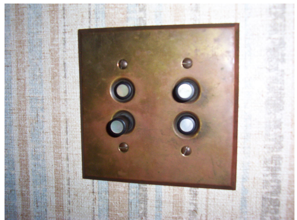
Early 1900s push-button light switches
