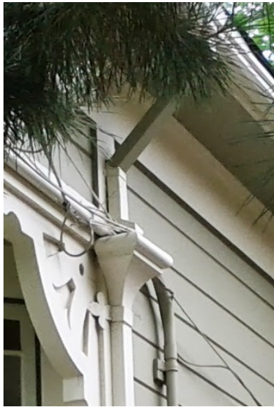
Conductor box on north corner downspout
