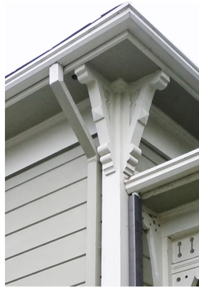
East corner downspout without conductor box
