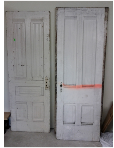
Two of the four replacement doors to be refurbished
