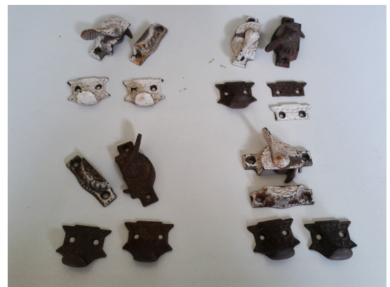
Eastlake-style window locks and sash pulls, believed to be original
