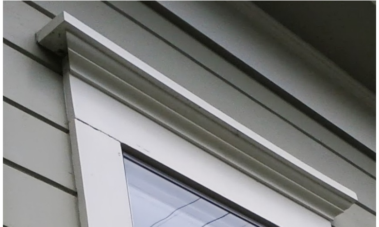
Bedroom window frame, with missing piece at top left
